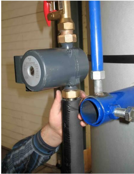
12. Connect the upper flexible pipe to the pump.
